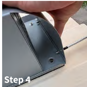
Step 4 Remainder of external hood is fastened.
