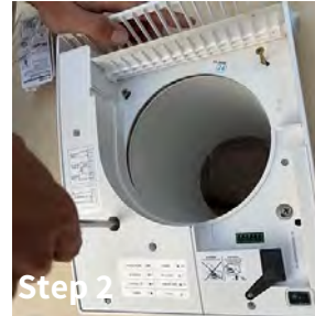
Step 2 Insert PVC pipe and fasten internal cover.
