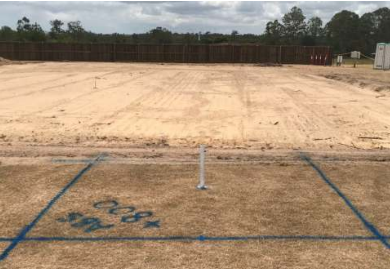
Secondary Wastewater Treatment System Ground Mark out
