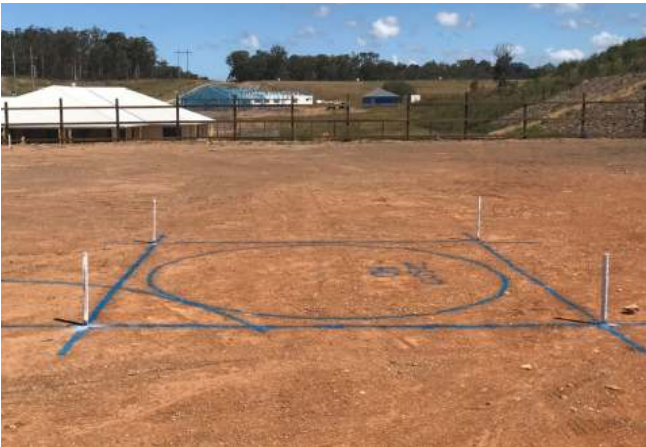
Rainwater System Ground Mark out
