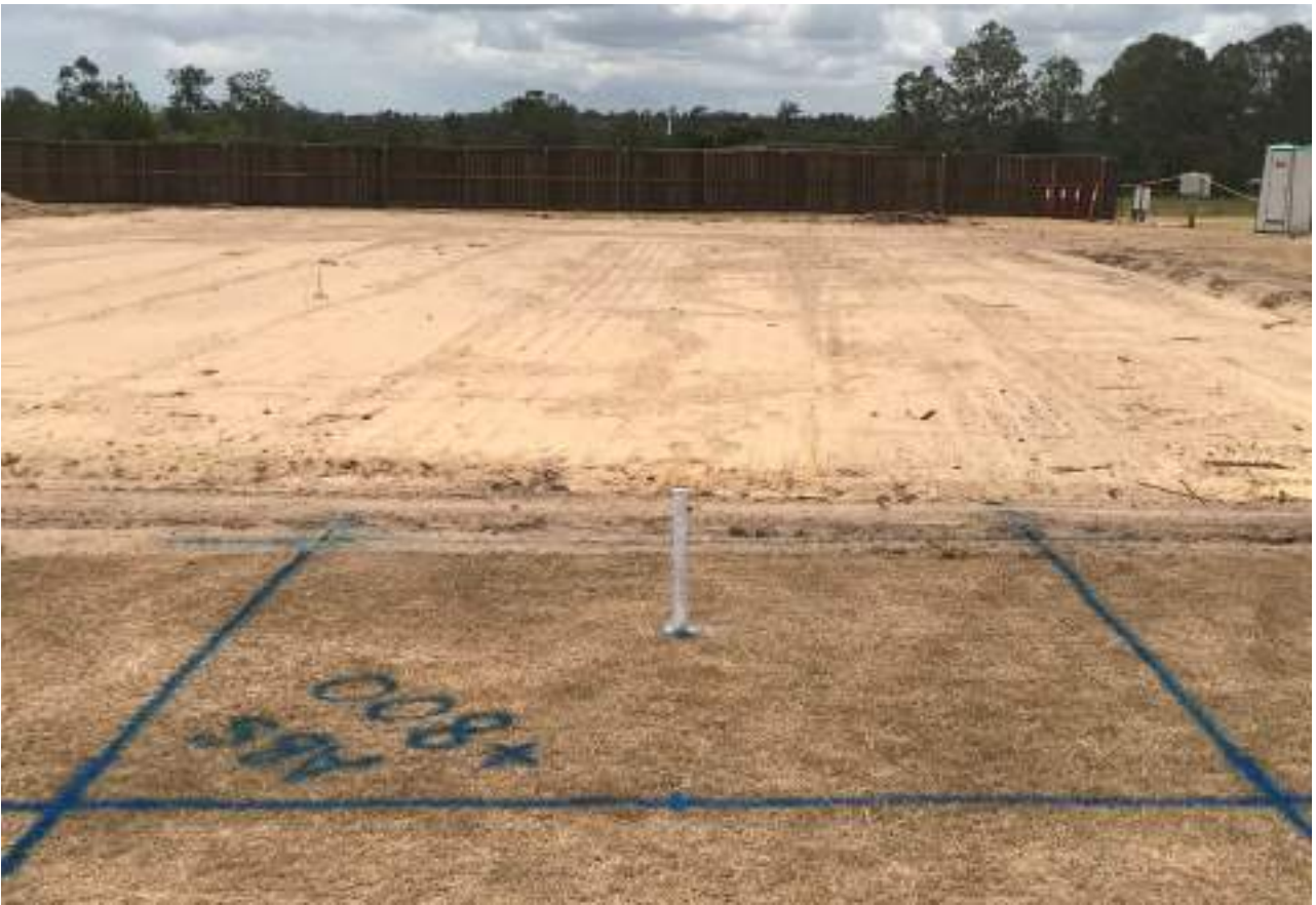
Secondary Wastewater Treatment System Ground Mark out
