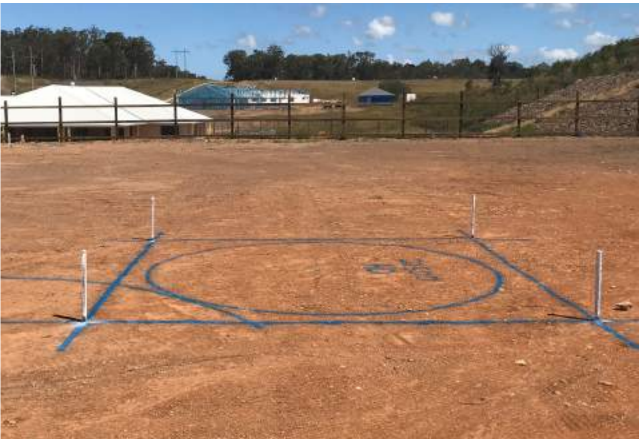
Rainwater System Ground Mark out
